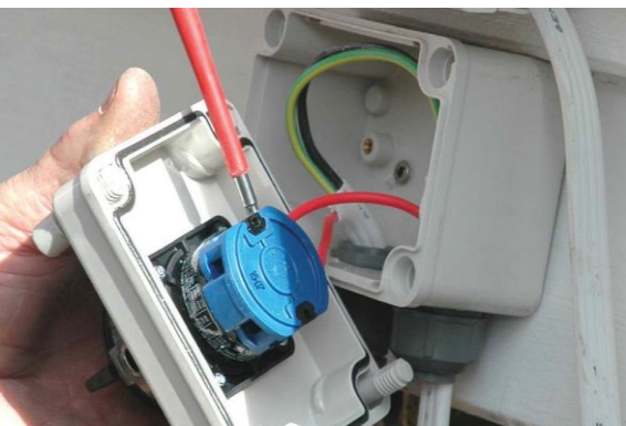
Figure 77: Install lockable isolating switch (B)
