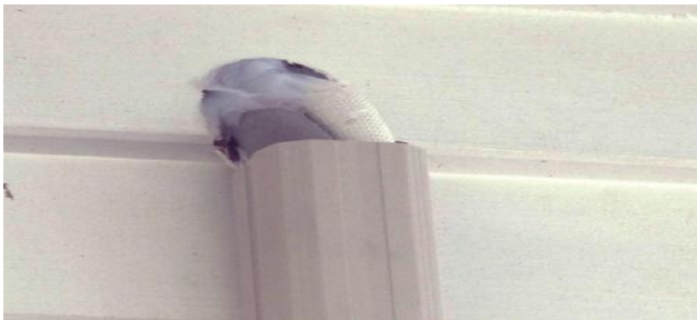
Figure 64: Fill hole around piping with sealant
