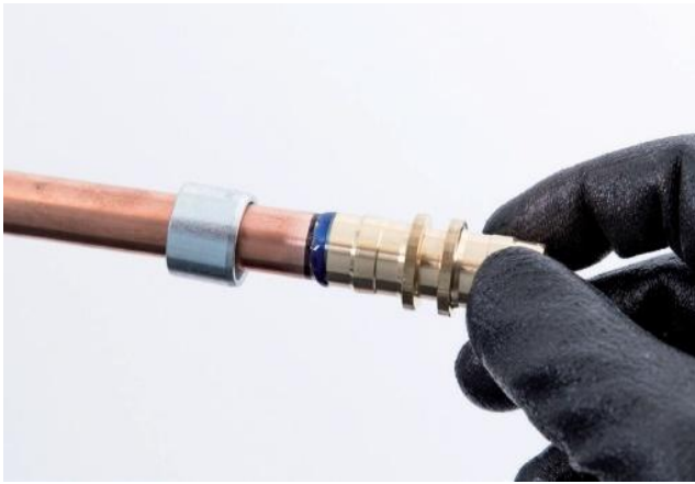
Figure 23: Step 7 – fitting connector
