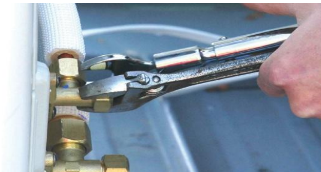
Figure 69: Tighten flare nut connections
