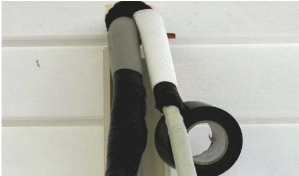
Figure 61: Tape drainage hose to drainage outlet
