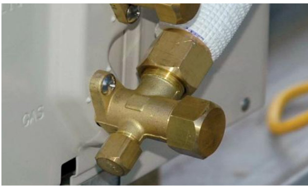
Figure 74: Tighten valve caps
