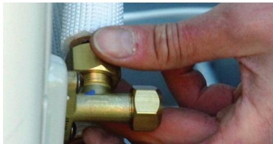
Figure 38: Connect the pipes (B)
