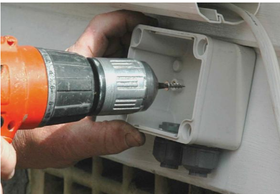
Figure 77: Install lockable isolating switch (B)
