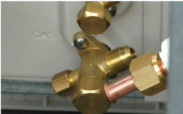
Figure 68: Connect pipes and tighten flare nut
