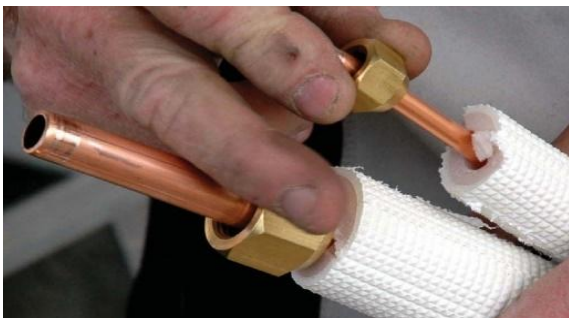
Figure 32: Flare the end of the tube (A)
