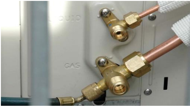
Figure 70: Remove vacuum pump and gauges (A)
