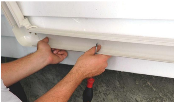
Figure 62: Install trunking neatly
