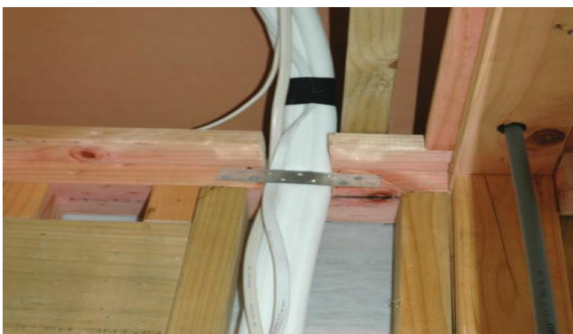
Figure 48: Fix galvanised mild steel strap to hold pipe and connection cable
