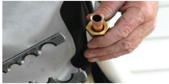
Figure 34: Flare the end of the tube (C)
