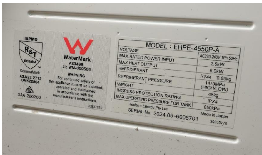
Figure 80: Example of nameplate on an outdoor unit
