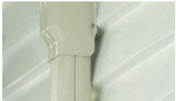
Figure 66: Fit cover over opening
