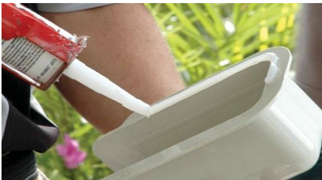
Figure 65: Seal around cover
