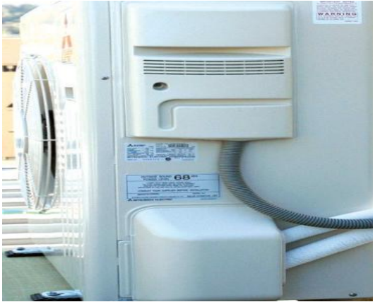
Figure 79: Replace service cover to outdoor unit
