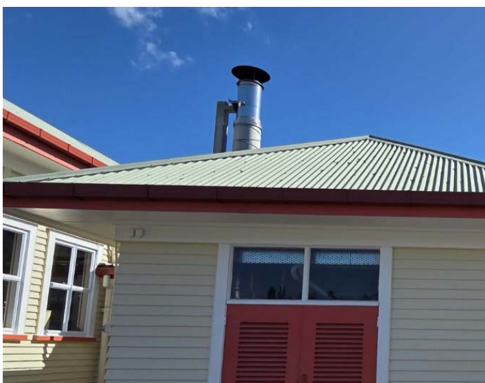
Boiler House Flue Stack
