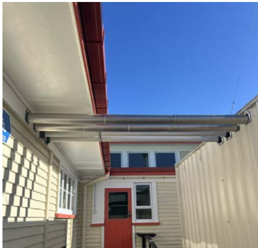
Pellet Transfer Lines & Hot Water Flow and Return Lines
