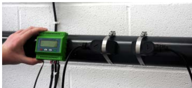
Figure 4: Example Ultrasonic Clamp-on Heat Meter
