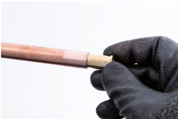
Figure 19: Step 3 – fitting insert when required to support pipe
