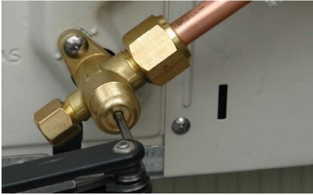
Figure 73: Progressively release the vacuum
