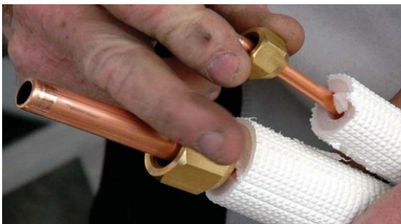
Figure 32: Flare the end of the tube (A)
