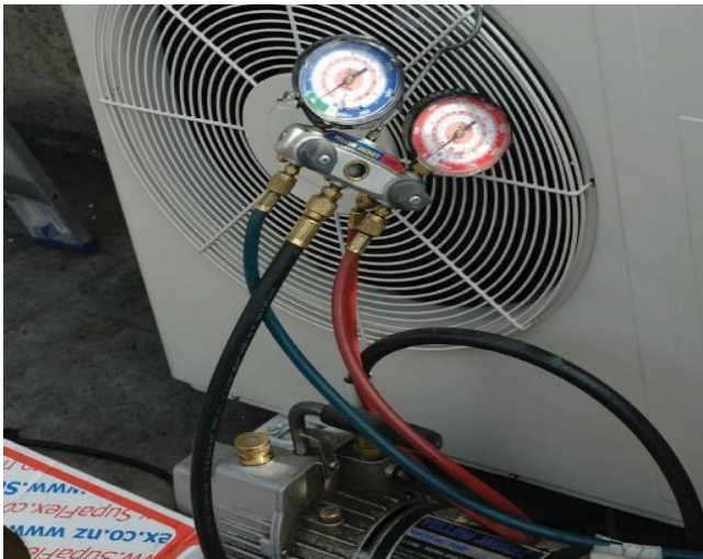
Figure 71: Remove vacuum pump and gauges (B)
