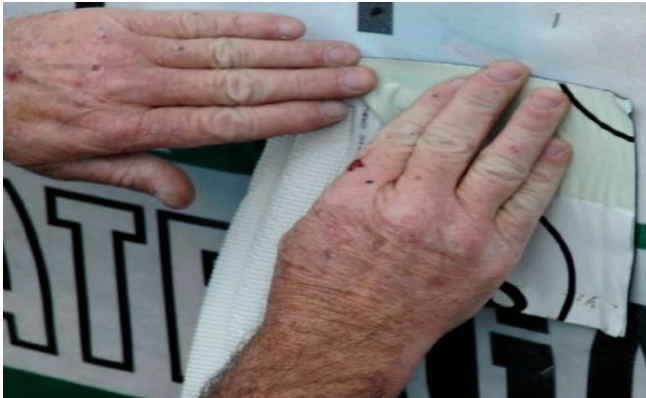
Figure 50: Seal pipes or sleeve
