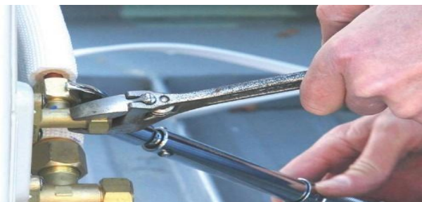
Figure 39: Tighten connection (A)
