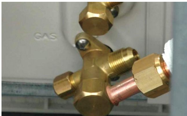
Figure 68: Connect pipes and tighten flare nut
