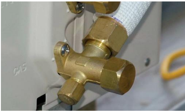
Figure 74: Tighten valve caps
