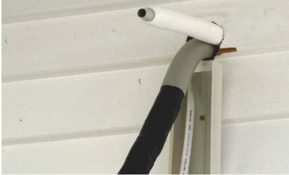
Figure 60: Bind insulation with vinyl tape
