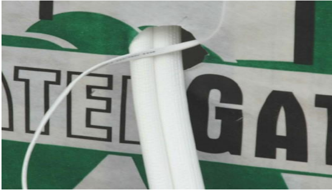
Figure 49: Feed pipe and cable through building wrap
