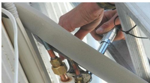
Figure 40: Tighten connection (B)
