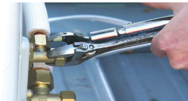
Figure 69: Tighten flare nut connections
