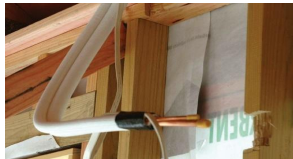
Figure 44: Notch top plate and studs (B)
