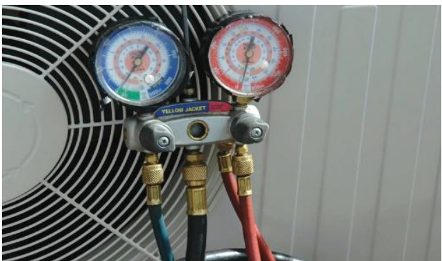
Figure 72: Remove vacuum pump and gauges (C)
