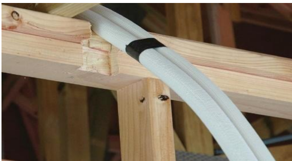
Figure 43: Notch top plate and studs (A)
