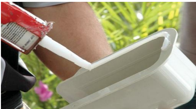
Figure 65: Seal around cover
