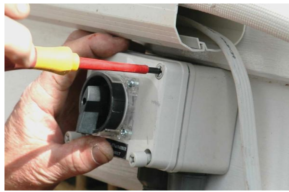
Figure 78: Install lockable isolating switch (C)
