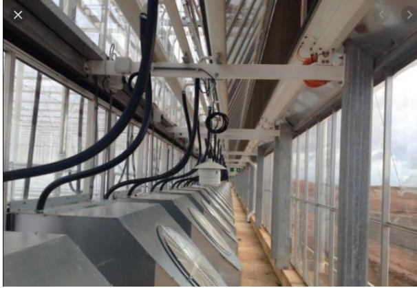
Fig. Interior of the air treatment corridor of an Ultra-Clima greenhouse from KUBO (NLD). Outside air can enter from the top and mixed with greenhouse air. The conditioned air is sucked into the grey boxes. Each grey box is an entrance to a sleeve. This is at D’Vine Ripe in South Australia. Source: www.aabnl.nl/en/project/68/ultra-clima-kas-voor-dvine-ripe.htm
