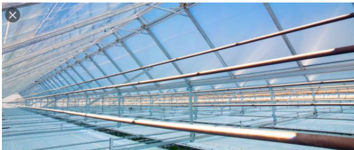
Fig. a black pipe filled with water receive a concentrated bundle of sunlight
