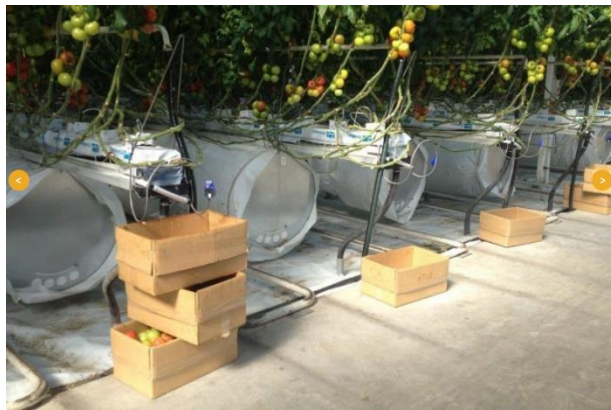
Fig. Interior of the air treatment corridor of an Ultra-Clima greenhouse from KUBO (NLD). Outside air can enter from the top and mixed with greenhouse air. The conditioned air is sucked into the grey boxes. Each grey box is an entrance to a sleeve. This is at D’Vine Ripe in South Australia. Source: www.aabnl.nl/en/project/68/ultra-clima-kas-voor-dvine-ripe.htm
