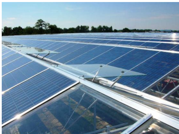
Hortisolar panels in Italy, solar roof, 2MW.
