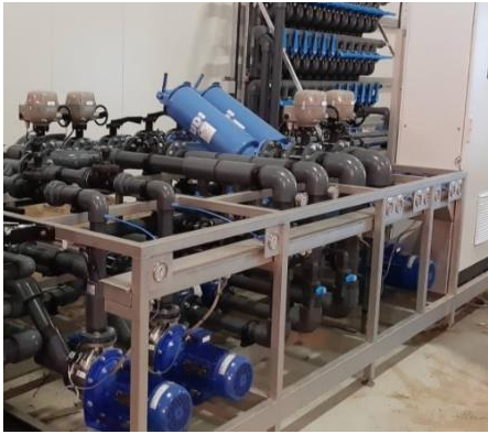
Photo left: installation for underground heat storage at Duijvestijn Tomaten (©Trees Borkus Henskens)
