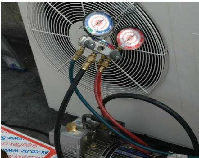
Figure 71: Remove vacuum pump and gauges (B)
