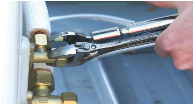
Figure 69: Tighten flare nut connections
