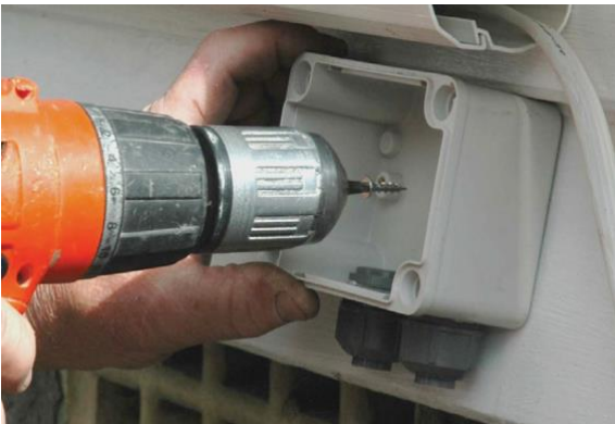
Figure 76: Install lockable isolating switch (A)
