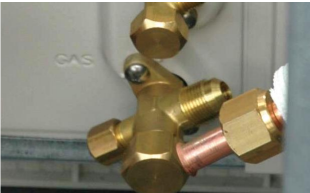
Figure 68: Connect pipes and tighten flare nut
