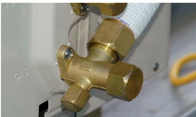
Figure 74: Tighten valve caps
