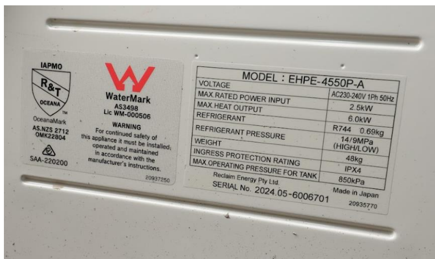
Figure 80: Example of nameplate on an outdoor unit
