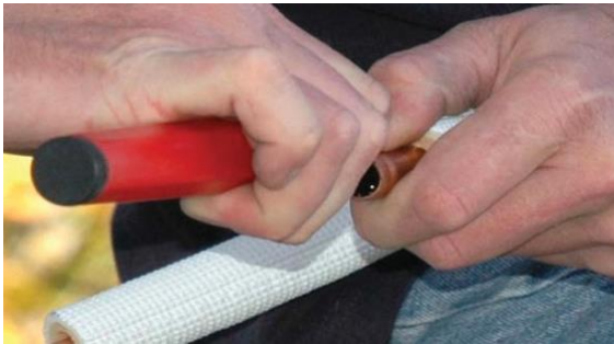
Figure 31: Place the flare nut over the pipe end
