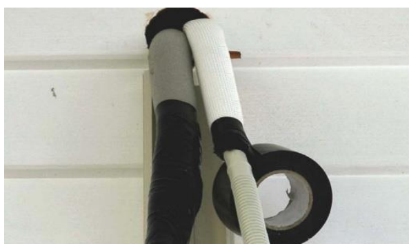
Figure 61: Tape drainage hose to drainage outlet
