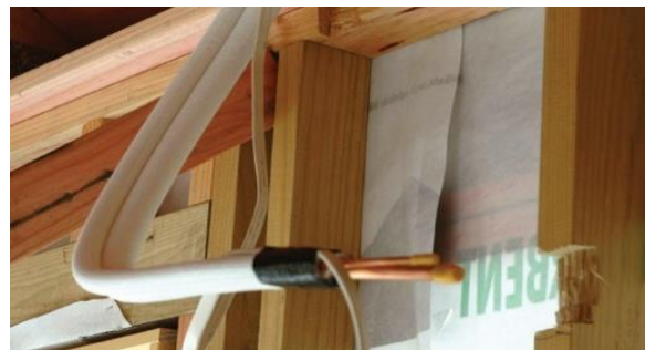
Figure 44: Notch top plate and studs (B)
