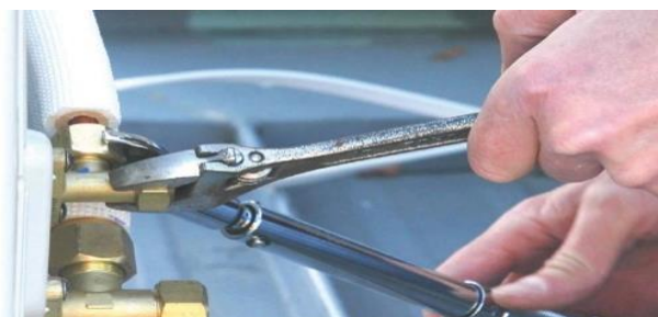
Figure 39: Tighten connection (A)
