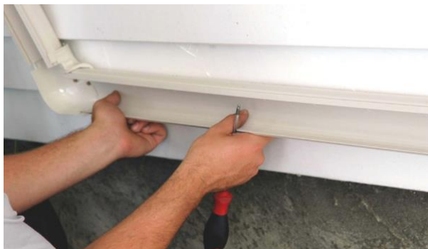
Figure 62: Install trunking neatly
