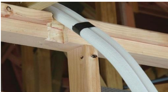
Figure 43: Notch top plate and studs (A)
