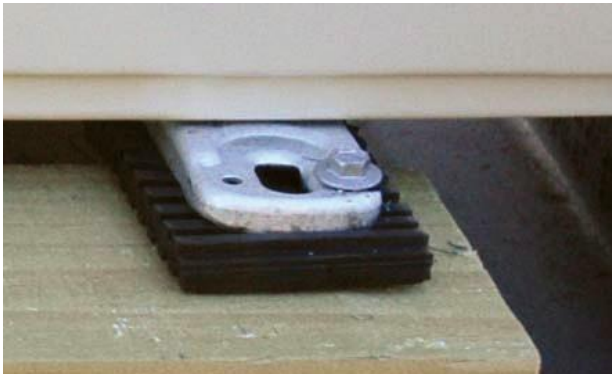
Figure 56: Pack with plastic shims to level
