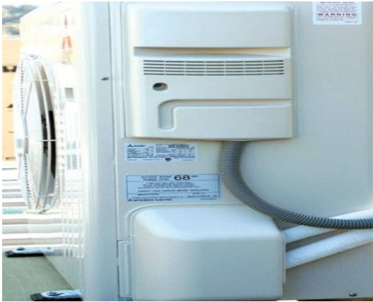
Figure 79: Replace service cover to outdoor unit
