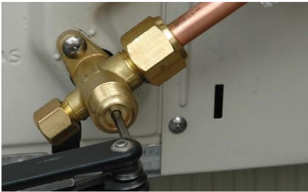
Figure 73: Progressively release the vacuum
