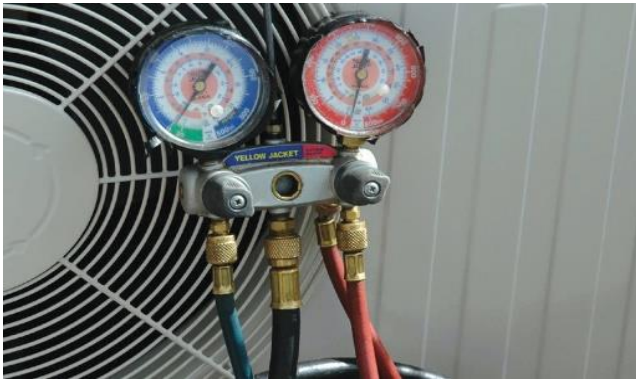
Figure 72: Remove vacuum pump and gauges (C)
