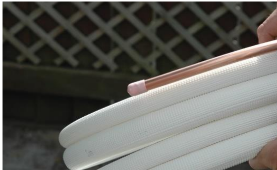
Figure 27: Cover pipe ends
