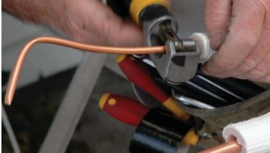
Figure 29: Cut pipe with tube cutters
