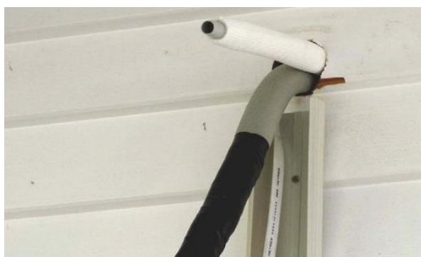
Figure 60: Bind insulation with vinyl tape
