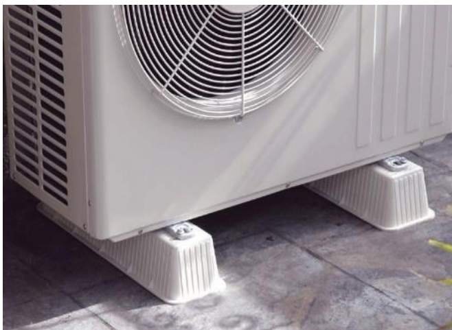
Figure 53: Unobstructed gap under outdoor unit fixed on concrete pad cast in place
