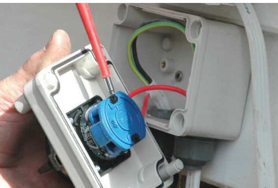
Figure 77: Install lockable isolating switch (B)
