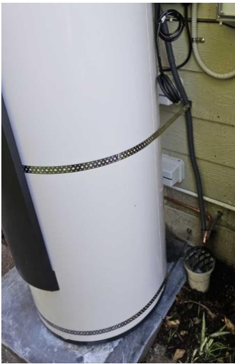
Figure 41: Condensate drain
