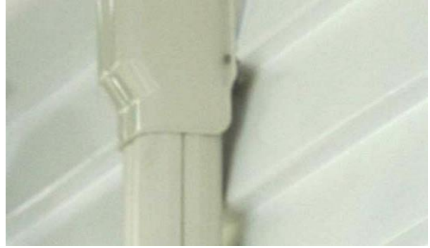
Figure 66: Fit cover over opening
