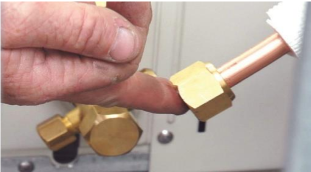
Figure 67: Apply oil to the back of the flare and the outdoor unit
