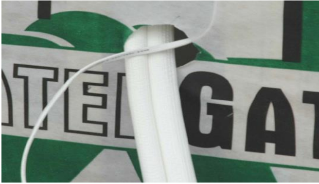
Figure 49: Feed pipe and cable through building wrap
