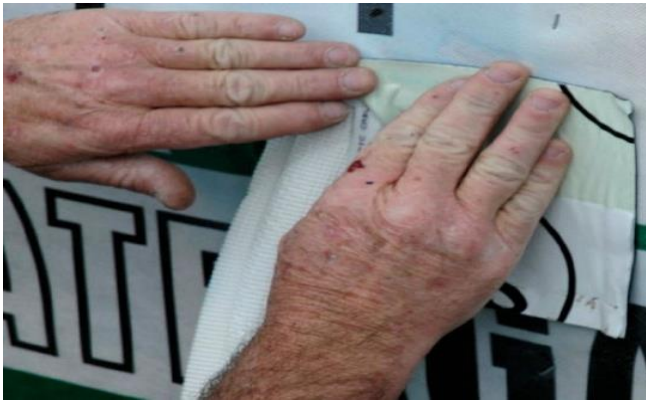
Figure 50: Seal pipes or sleeve
