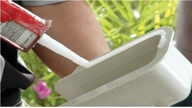
Figure 65: Seal around cover
