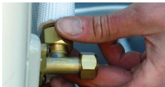
Figure 38: Connect the pipes (B)
