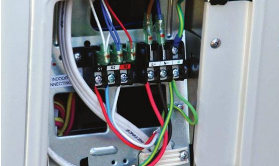
Figure 75: Connect power supply cable to terminal block
