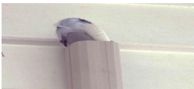
Figure 64: Fill hole around piping with sealant
