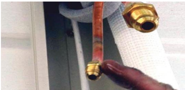
Figure 36: Apply oil to the back of the flared pipe and the flare joint
