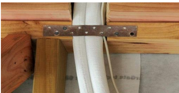
Figure 45: Fix galvanised mild steel strap to hold pipe and cable
