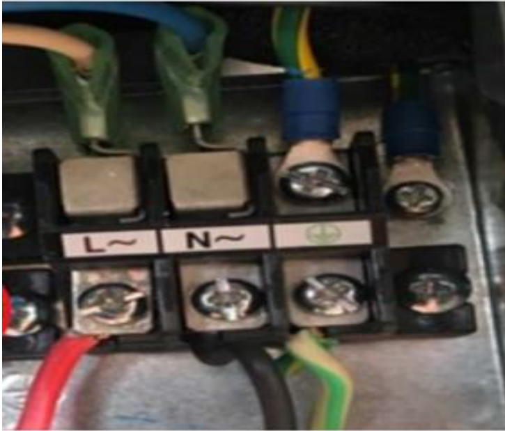
Figure 81: Typical wiring connections
