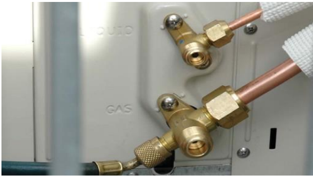
Figure 70: Remove vacuum pump and gauges (A)
