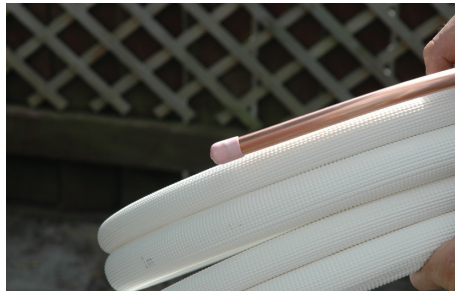
Figure 6.12 Cover pipe ends
