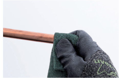
Figure 6.3 Step 2: Roughing the end surface
