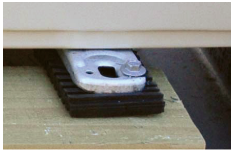
Figure 7.17 Pack with plastic shims to level
