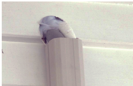
Figure 7.23 Fill hole around piping with sealant
