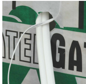
Figure 6.33 Feed pipe/cables through building wrap
