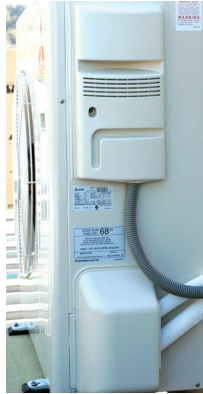
Figure 9.5 Replace service cover to outdoor unit
