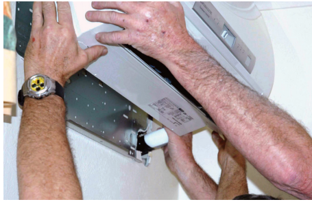
Figure 7.9 Attach unit to wall bracket (A)
