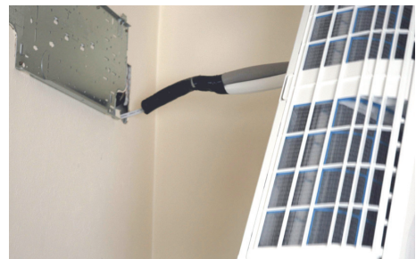
Figure 7.8 Feed taped bundle through the hole
