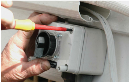
Figure 9.4 Install lockable isolating switch (C)
