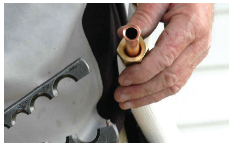
Figure 6.19 Flare the end of the tube (C)
