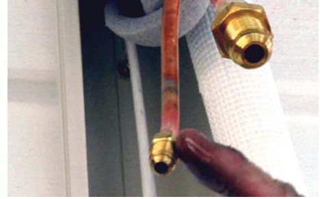
Figure 6.21 Apply oil to the back of the flared pipe and the flare joint
