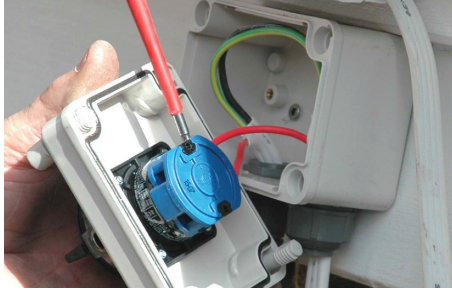
Figure 9.4 Install lockable isolating switch (C)
