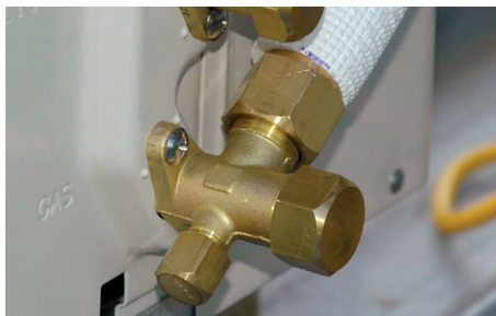
Figure 7.33 Tighten valve caps
