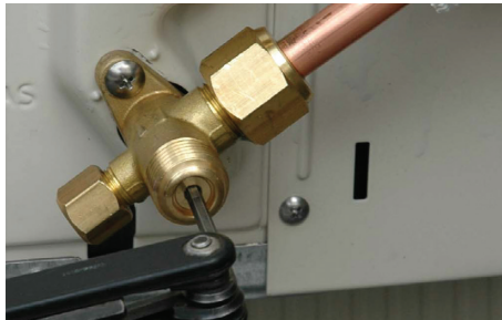
Figure 7.32 Progressively release the vacuum
