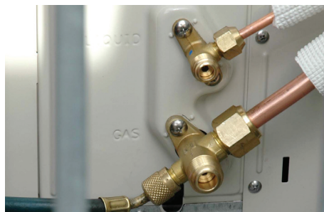
Figure 7.29 Remove vacuum pump and gauges (A)
