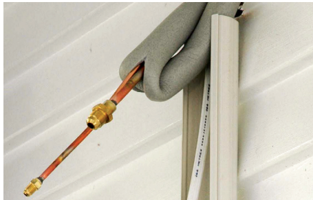
Figure 7.13 Expose flared pipe ends
