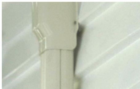
Figure 7.25 Fit cover over opening
