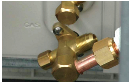
Figure 7.27 Connect pipes and tighten flare nut
