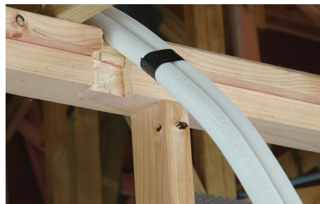
Figure 6.27 Notch the top plate and studs (A)
