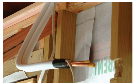
Figure 6.28 Notch the top plate and studs (B)
