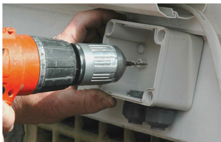
Figure 9.2 Install lockable isolating switch (A)
