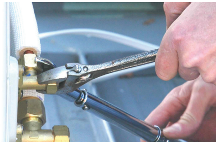
Figure 6.24 Tighten connection (A)
