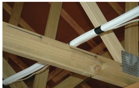
Figure 6.26 Run pipe/cable across truss chord/ceiling joist
