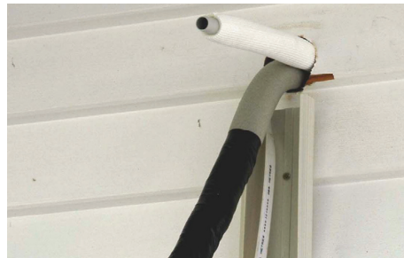
Figure 7.19 Bind insulation with vinyl tape
