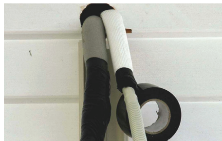
Figure 7.20 Tape drainage hose to drainage outlet
