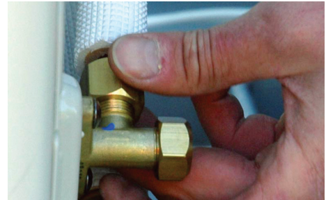
Figure 6.23 Connect the pipes (B)
