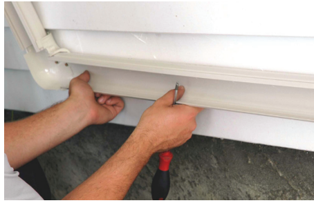
Figure 7.21 Install trunking neatly
