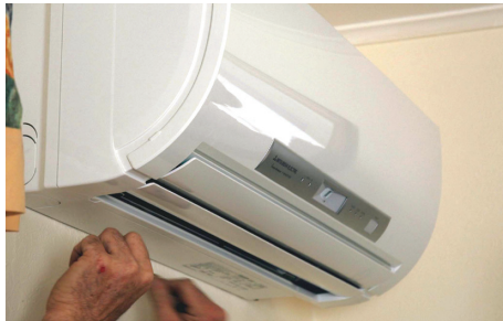
Figure 7.11 Ensure unit is securely seated
