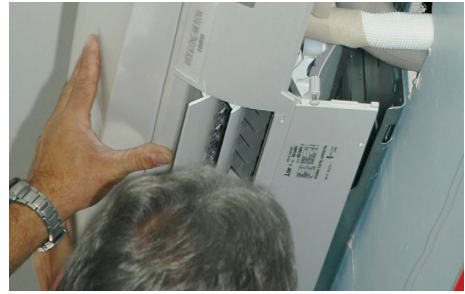
Figure 7.10 Attach unit to wall bracket (B)
