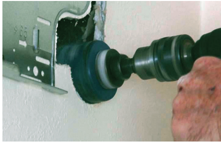
Figure 7.3 Drill a hole through the wall
