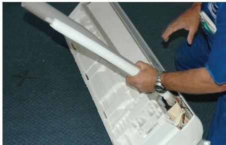
Figure 7.5 Release the tubing and drainage hose
