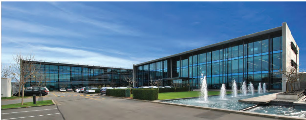
Image: 14 Show Place, Christchurch headquarters for IAG and owned by Goodman Property. A collaboration between landlord and tenant delivered a building with leading-edge energy credentials – a 5 star “market leading” rating.
