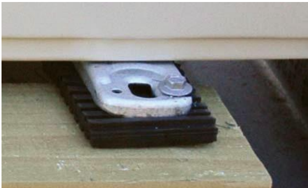
Figure 57: Pack with plastic shims to level
