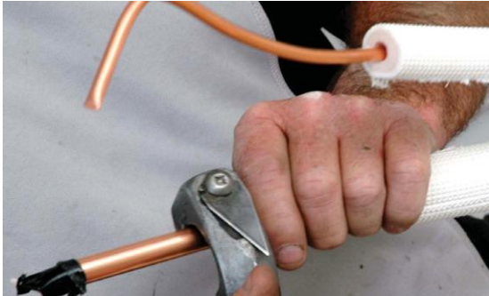
Figure 26: Pipe opening facing down when cutting
