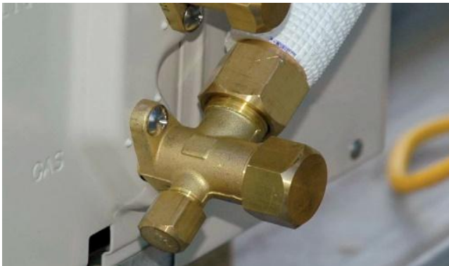
Figure 74: Tighten valve caps
