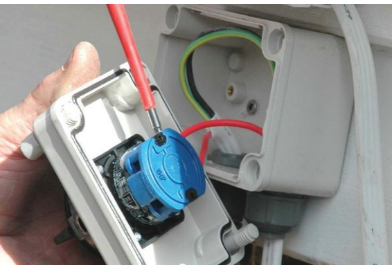
Figure 77: Install lockable isolating switch (B)
