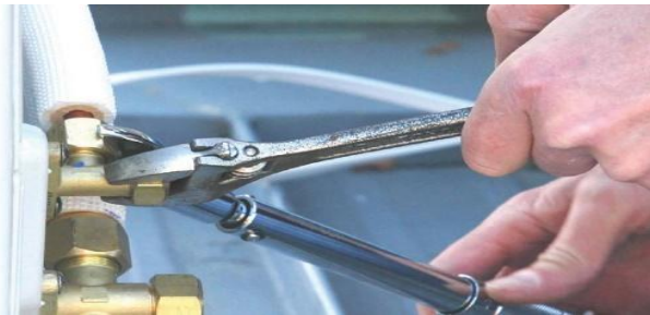
Figure 39: Tighten connection (A)
