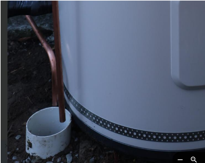
Figure 51: TPR drain
