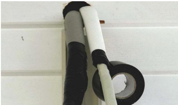
Figure 61: Tape drainage hose to drainage outlet
