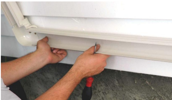
Figure 62: Install trunking neatly
