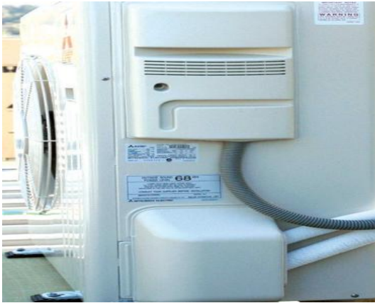
Figure 79: Replace service cover to outdoor unit
