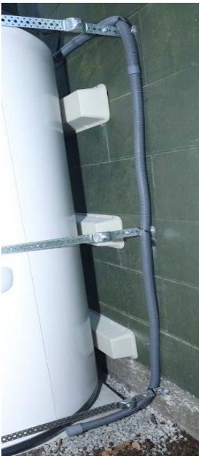
Figure 41: Condensate drain
