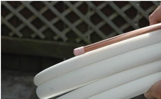
Figure 27: Cover pipe ends
