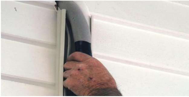
Figure 63: Fit refrigerant piping, drainage pipe and connecting cable into trunking
