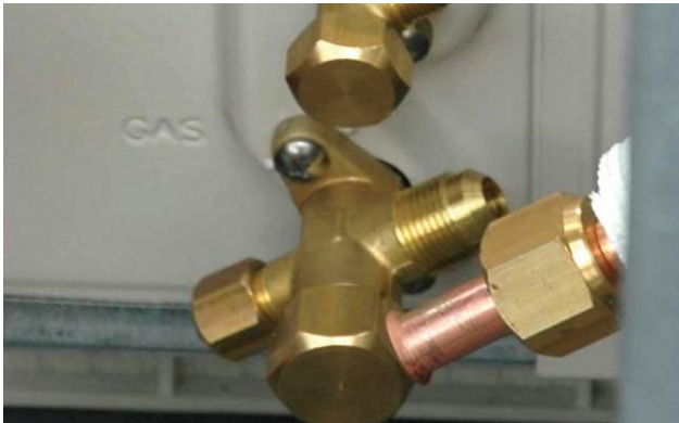
Figure 68: Connect pipes and tighten flare nut
