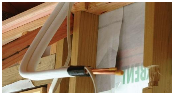
Figure 44: Notch the top plate and studs (B)
