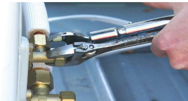
Figure 69: Tighten flare nut connections
