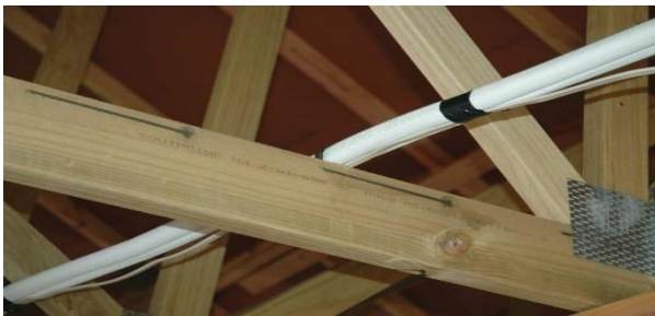
Figure 42: Run pipe/cable across truss chord/ceiling joist
