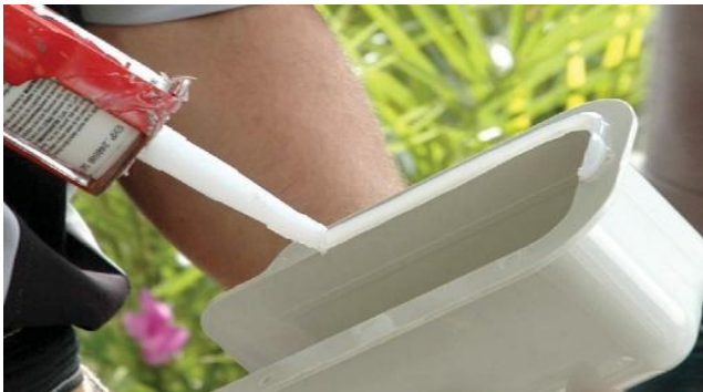
Figure 65: Seal around cover
