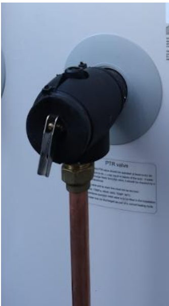
Figure 52: TPR valve and vertical discharge pipe
