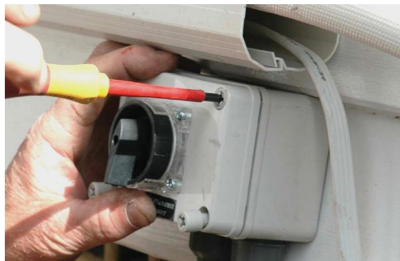
Figure 78: Install lockable isolating switch (C)
