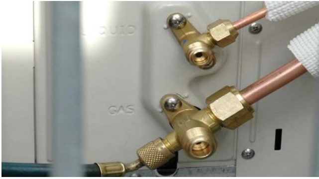
Figure 70: Remove vacuum pump and gauges (A)
