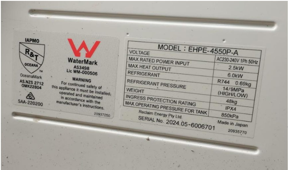
Figure 80: Example of a nameplate on an outdoor unit
