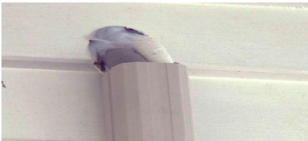
Figure 64: Fill hole around piping with sealant
