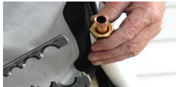
Figure 34: Flare the end of the tube (C)
