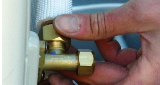
Figure 38: Connect the pipes (B)
