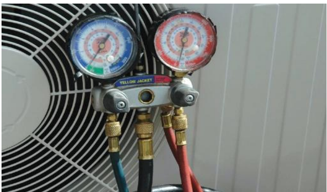
Figure 72: Remove vacuum pump and gauges (C)
