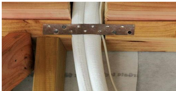
Figure 45: Fix galvanised mild steel strap to hold pipe/cable
