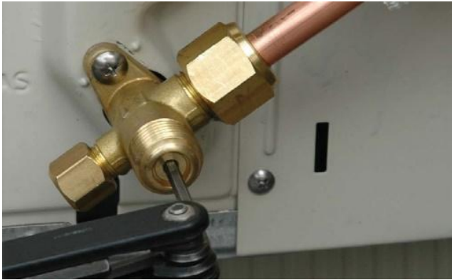
Figure 73: Progressively release the vacuum
