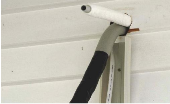
Figure 60: Bind insulation with vinyl tape
