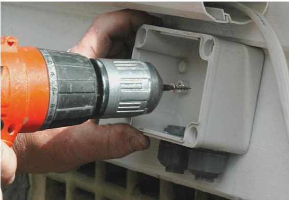
Figure 76: Install lockable isolating switch (A)
