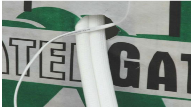
Figure 49: Feed pipe/cables through building wrap
