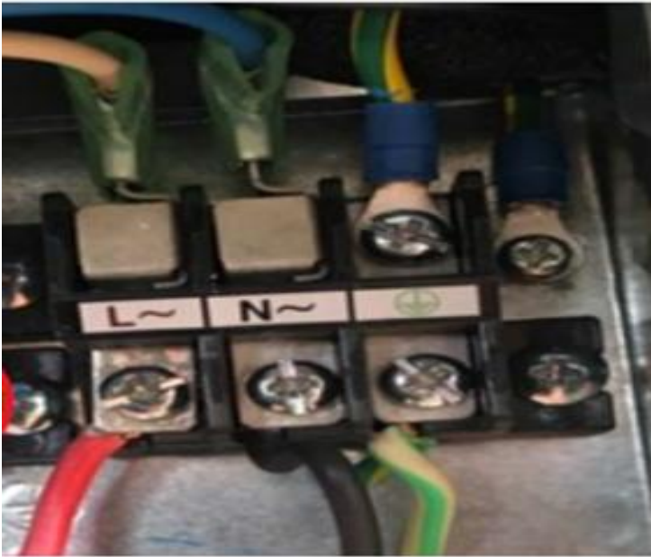
Figure 81: Typical wiring connections for an all-in-one system
