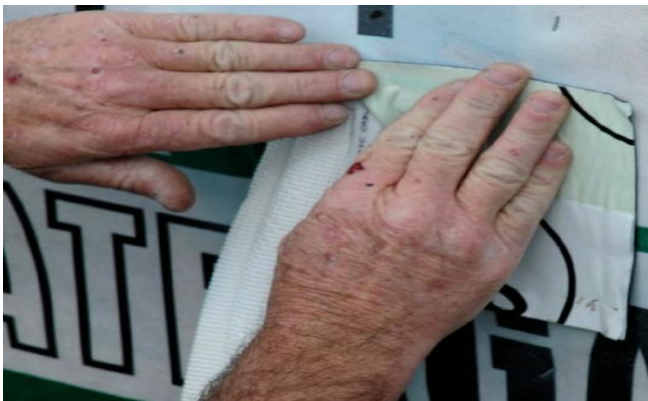
Figure 50: Seal pipes or sleeve
