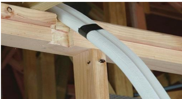
Figure 43: Notch the top plate and studs (A)
