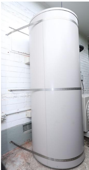
Figure 59: Seismic restraint for a hot water cylinder
