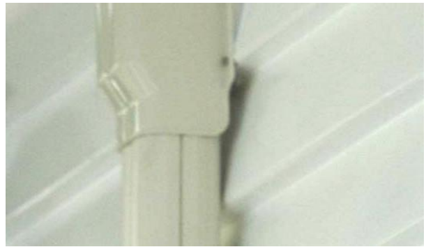
Figure 66: Fit cover over opening
