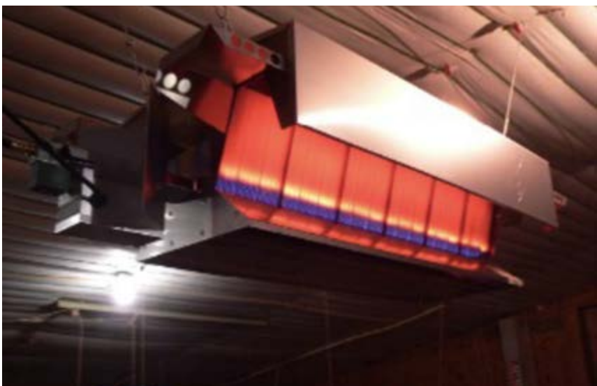
Rectangular open-flame radiant brooder Image credit: University of Kentucky
