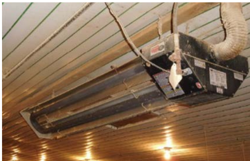
Closed-flame radiant tube brooder Image credit: University of Kentucky
