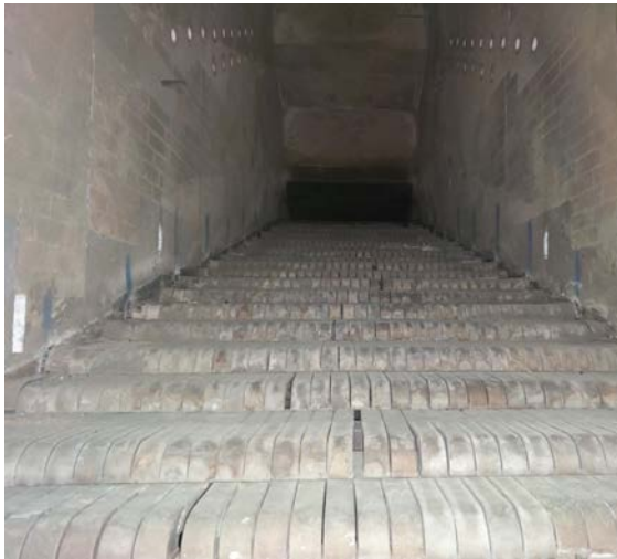
Figure 11: Boiler Grate Internal View
