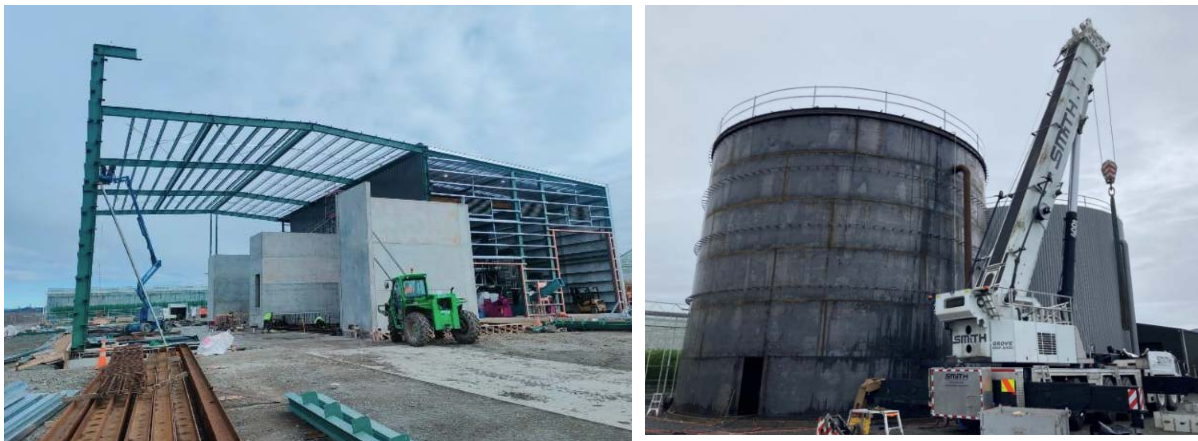
Figure 24: Installation of Boiler House & Thermal Storage Tanks
