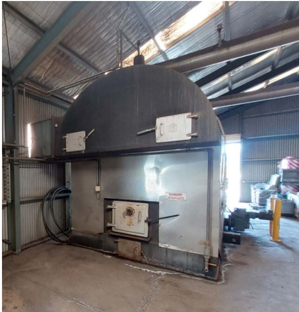
Figure 3: Example of Old Fire-tube Coal Boiler
