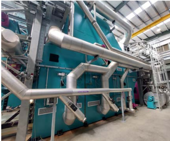
Figure 13: Primary Air and FGR Pipework
