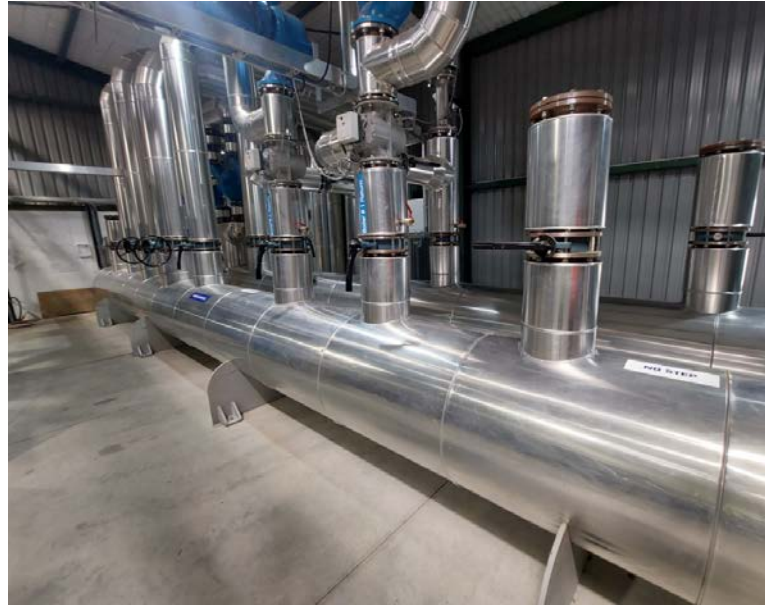
Figure 17: Hot and Cold-Water Headers
