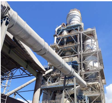
Figure 4: Suspension Preheater
