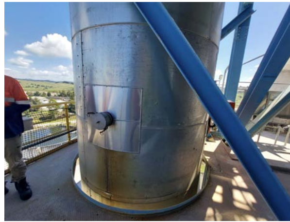
Figure 7: Emissions Testing Ports
