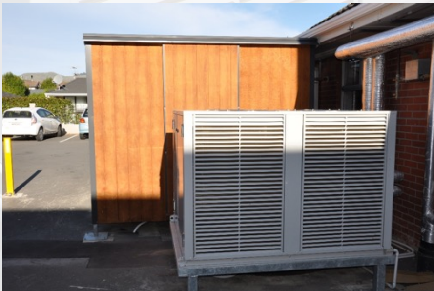
Decarbonised Energy Solutions' Domestic Hot Water Module for reticulated hot water service
