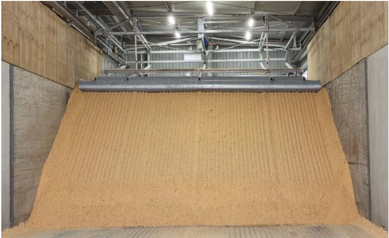
Figure 4: Example of Toploader showing Trolley System (not Waitoa)
