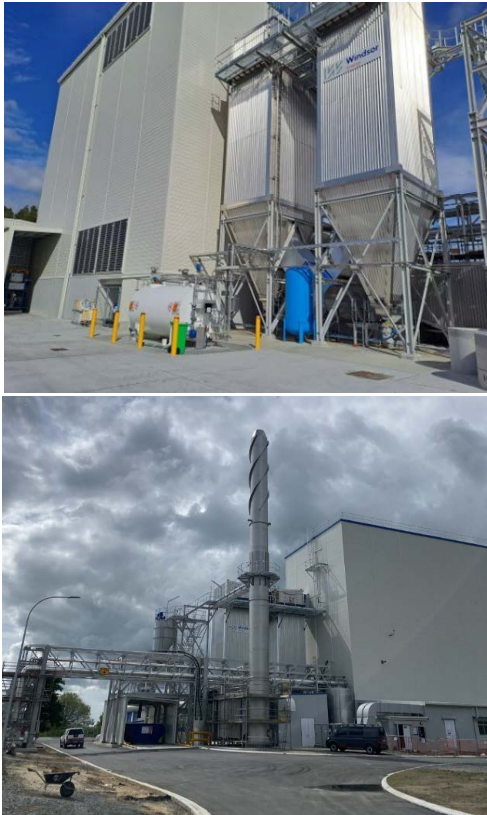
Figure 23: External View of Baghouse, Flue, Boiler and Pipebridge
