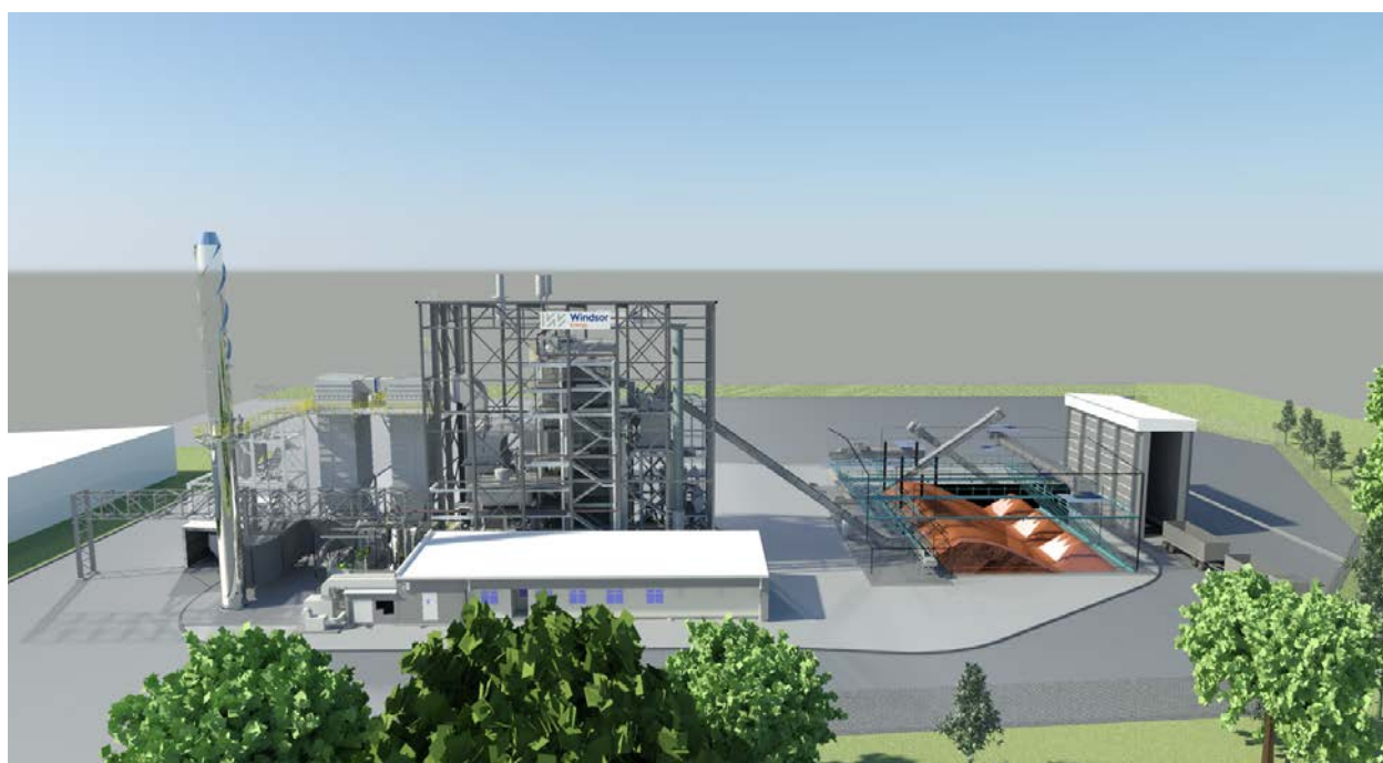
Figure 2: Bubbling Fluidised Bed Boiler (left) & Biomass Handling & Feed System (right)
