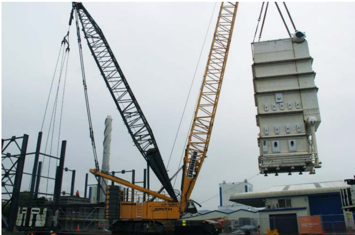
Figure 21: 110 Tonne Boiler Lift
