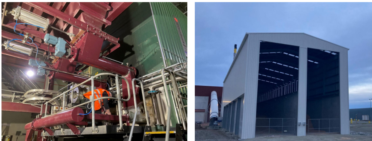
Figure 9: Biomass pneumatic feeder and fuel store at McCain Timaru
