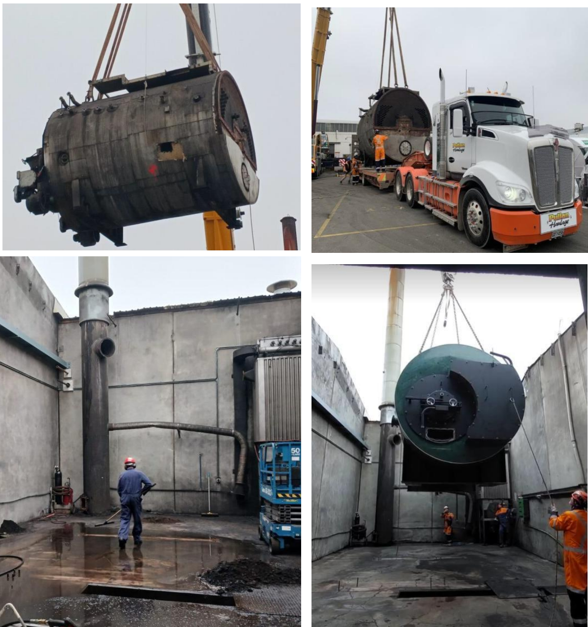
Figure 11: Old Boiler Removal and New Boiler Installation
