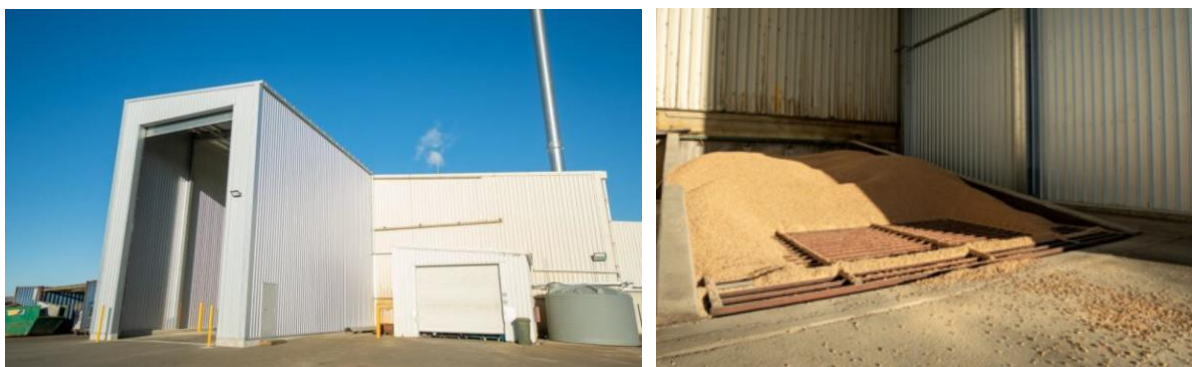
Figure 3: Wood Pellet & Chip Store at AlSCO Uniforms Invercargill
