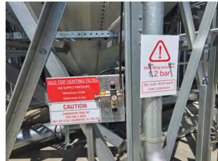
Maximum delivery pressure of 1.2 bar to prevent degrading pellet integrity
