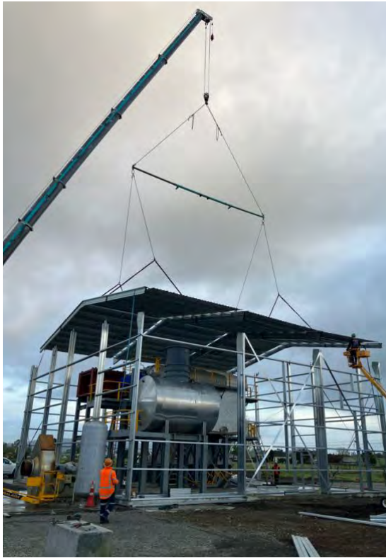
Crane lift of roof onto boiler house frame
