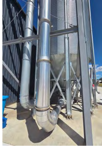
Silos showing, noise insulation on delivery tubes
