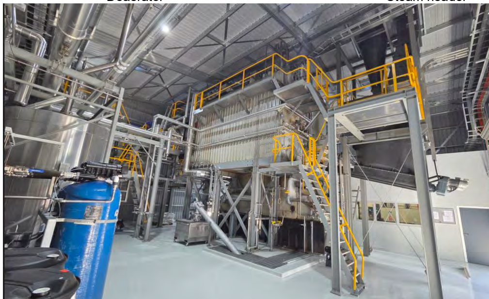
Maxitherm Steam Boiler
