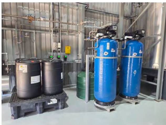
Water treatment: Softener, Spirax Sarco Alpha, Theta Gold, Omega Green
