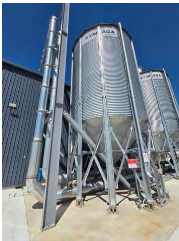
Silos showing, noise insulation on delivery tubes
