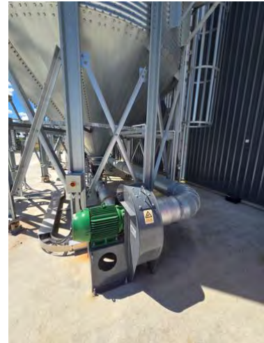
Air fan which blows pellets to boiler day hopper
