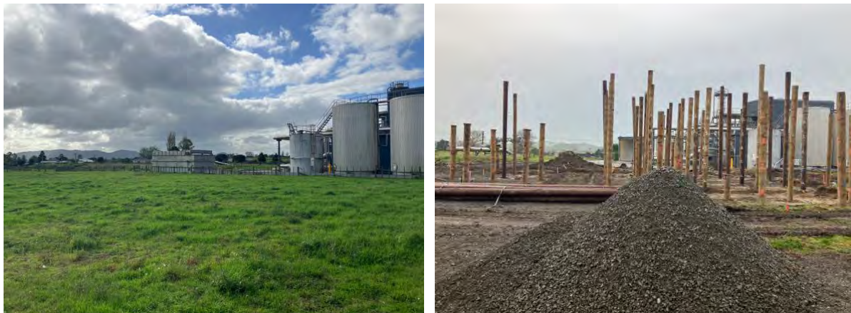
Figure 8: Selected Adjacent Site & Piled Foundation in Construction in July 2024
