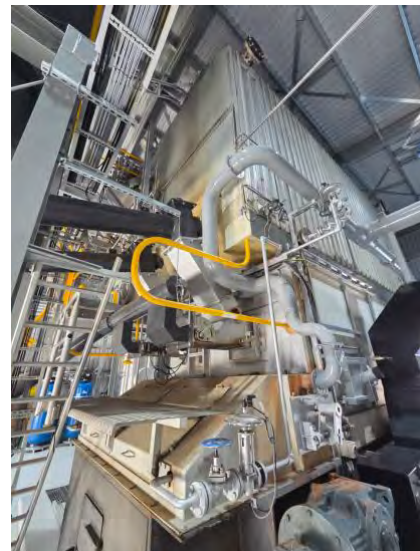
Air fan which blows pellets to boiler day hopper
