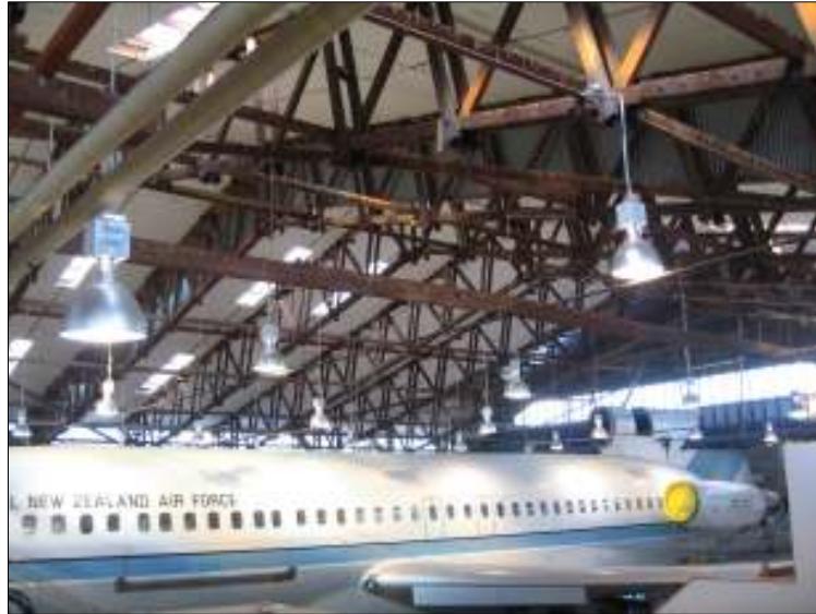
Lighting in Hangar No.4
