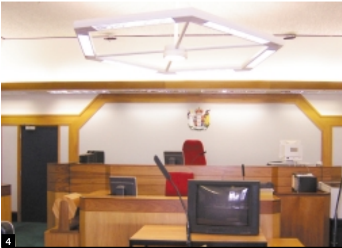
4 BIG SAVINGS ARE EXPECTED FROM INSTALLING SEPARATE AIR CONDITIONING CONTROLS FOR THE BUILDING'S 11 COURTROOMS SO ONLY THOSE IN USE ARE HEATED OR COOLED.
