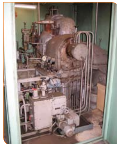
The steam turbine spins at 11,800 RPM and makes a noise similar to a jet airliner.
