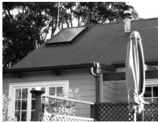
Figure 3: Flat-plate solar collector panel looking similar to a skylight (photo by Emsol)
