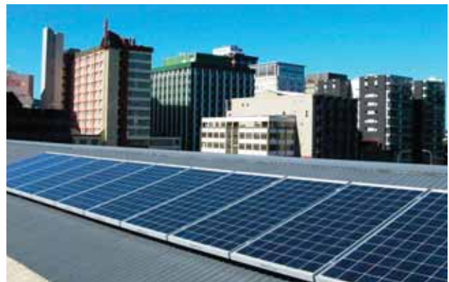
A PV panel installed at Clifton School, Wellington. Photo courtesy of Genesis Energy's Schoolgen programme.
