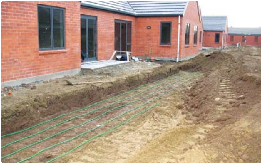
Installing the ground source heat pump's captors.
