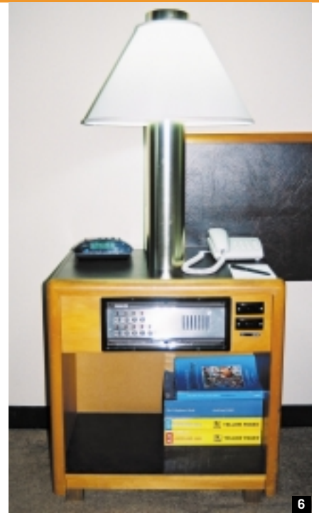
6 REPLACING 75 W INCANDESCENTS WITH 26 W COMPACT FLUORESCENTS IN THE CENTRA AUCKLAND AIRPORT HOTEL'S BEDSIDE LAMPS HAS IMPROVED OUTPUT.
