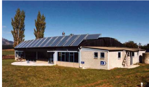
High school pool complex Otautau
