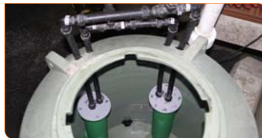
The two canisters encase the 6m, 20mm titanium Spirex heat exchangers – the heart of The Retriever.
