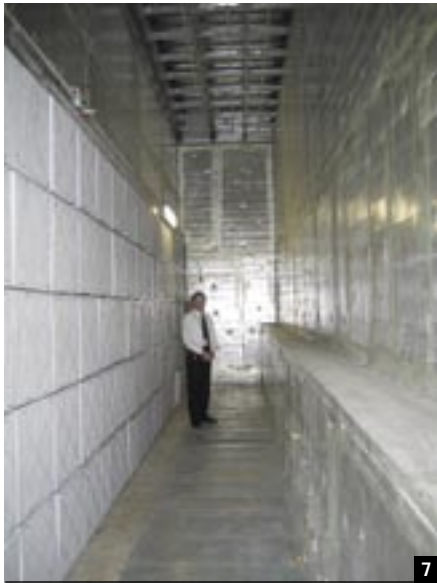
7 MIKE ANTHONY STANDS IN THE ENORMOUS DUCT FOR THE RETURN AIR, WHERE ALL THE BUILDING'S AIR IS PULLED DOWN TO BE FILTERED, REHEATED OR COOLED AND MIXED WITH FRESH OUTSIDE AIR TO RE-ENTER THE BUILDING. PRESSURE SENSORS CONTROL THE RETURN AIR FANS SO THEY USUALLY OPERATE AT 50% TO 70% OF THEIR CAPACITY. WELL-ADJUSTED CLOSE CONTROL AVOIDS ENERGY WASTE.
