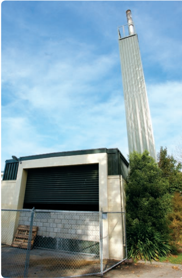
The new boilers produce five times less particulate emissions than the old coal-fire boilers.
