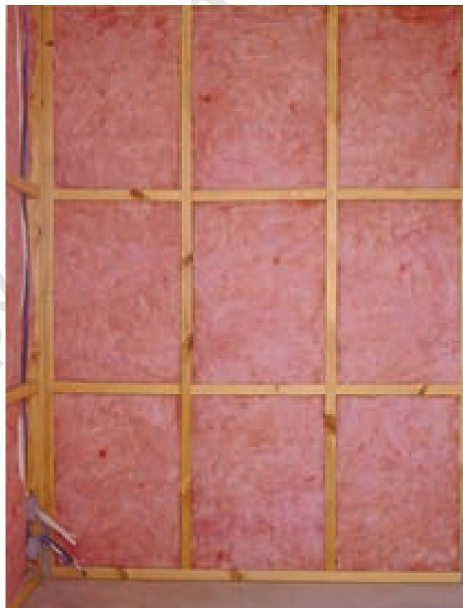
Figure 10 – Segments correctly installed in new wall
