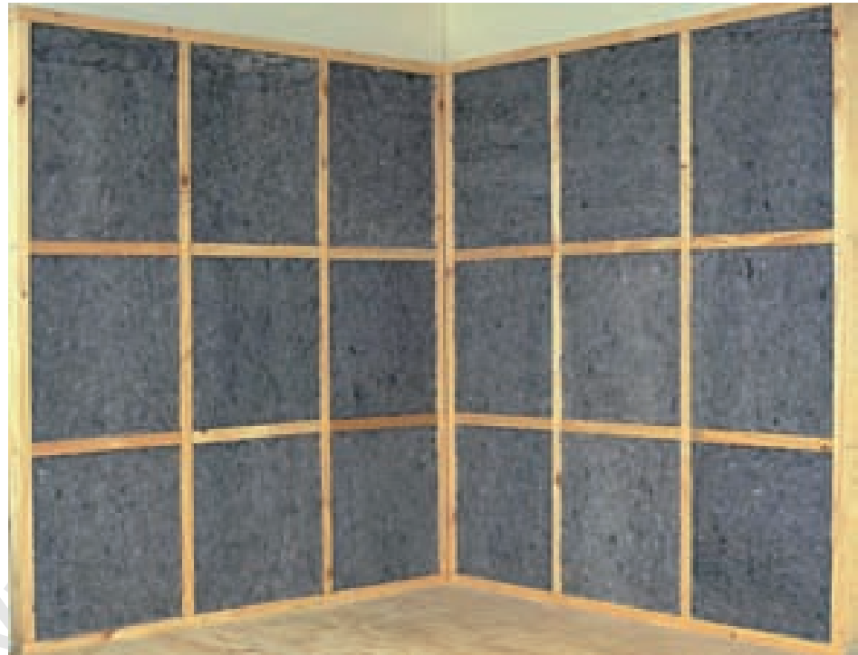
Figure 13 – Completed blanket installation in framed walls
