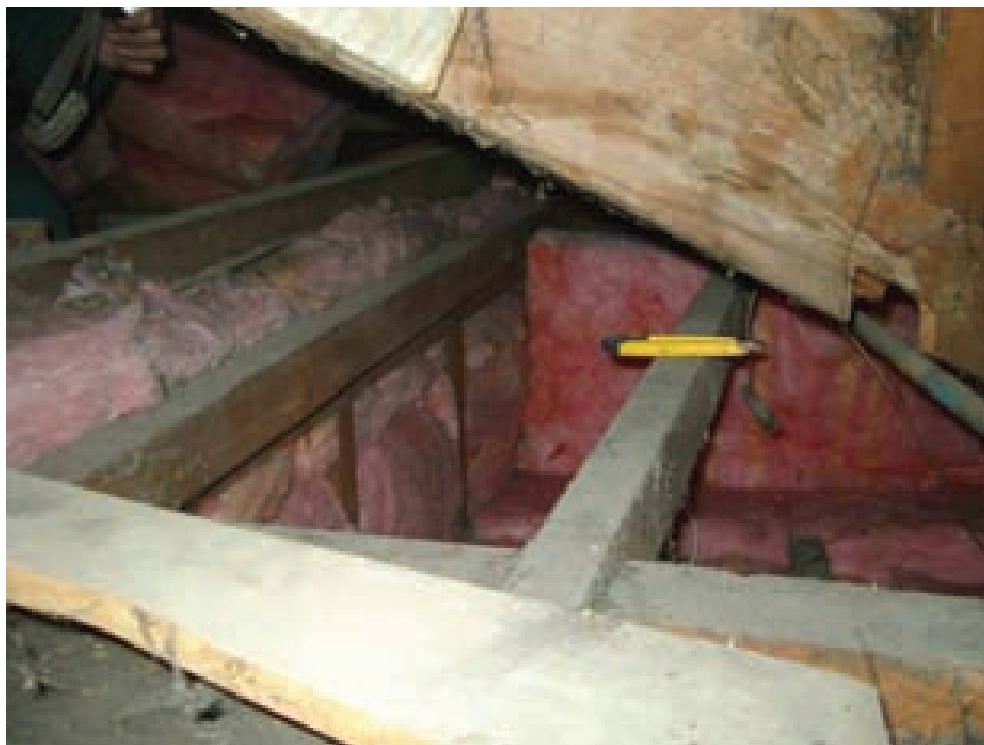
Figure 2 – Recessed ceiling space
