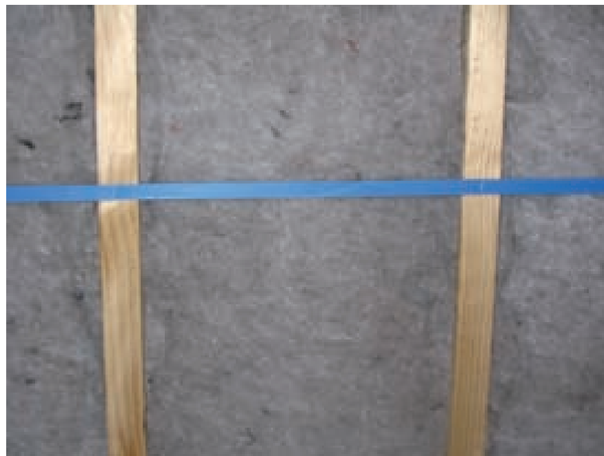
Figure 5 – Blanket in ceiling secured with strapping
