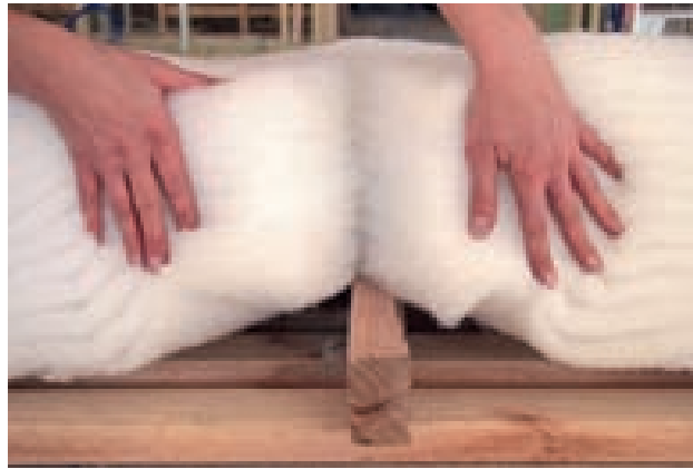
Figure 8 – Blanket torn over the ceiling joist 300mm back from the top plate
