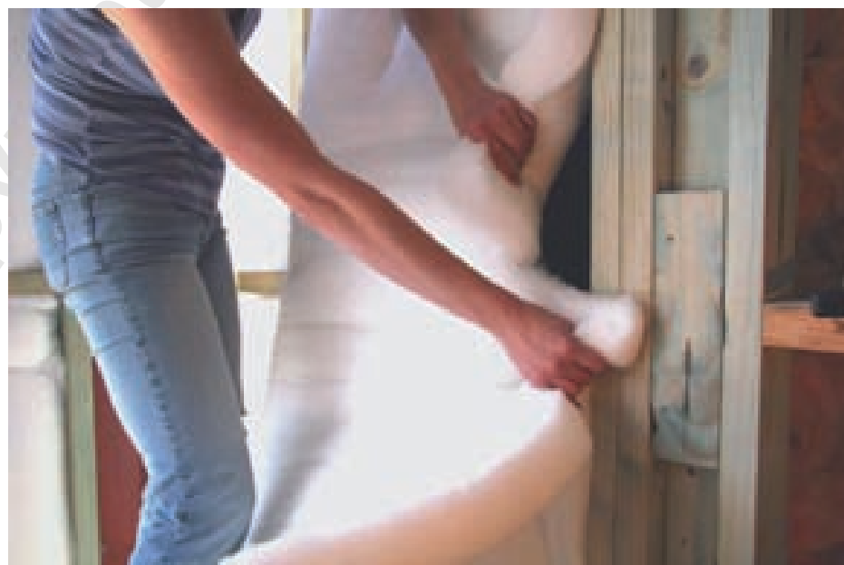
Figure 11 – Tearing blanket to fit
