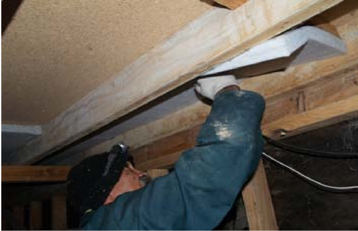
Figure 16 – Fitting semi-rigid sheets
