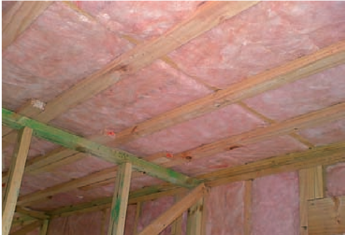
Figure 4 – Segments in unlined ceiling
