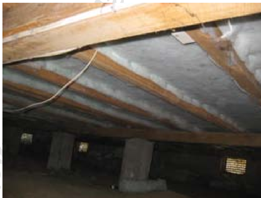
Figure 14 – Installing underfloor blanket
