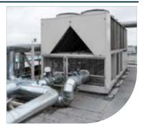
The heat recovery machine will transfer heat from the atmosphere to the heating system, and/or from the cooling system to the heating system, when necessary, using some energy from both sources simultaneously. This provides a very efficient solution for heating and cooling a building. 2-pipe machines can be arranged in banks to provide simultaneous heating and cooling from a group of machines.
